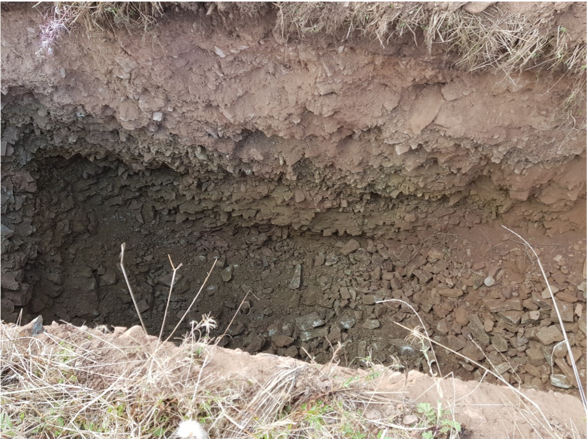
Number: TP21 Project Glounthaune Housing Phase 2 Project No P18170 Engineer AECOM
