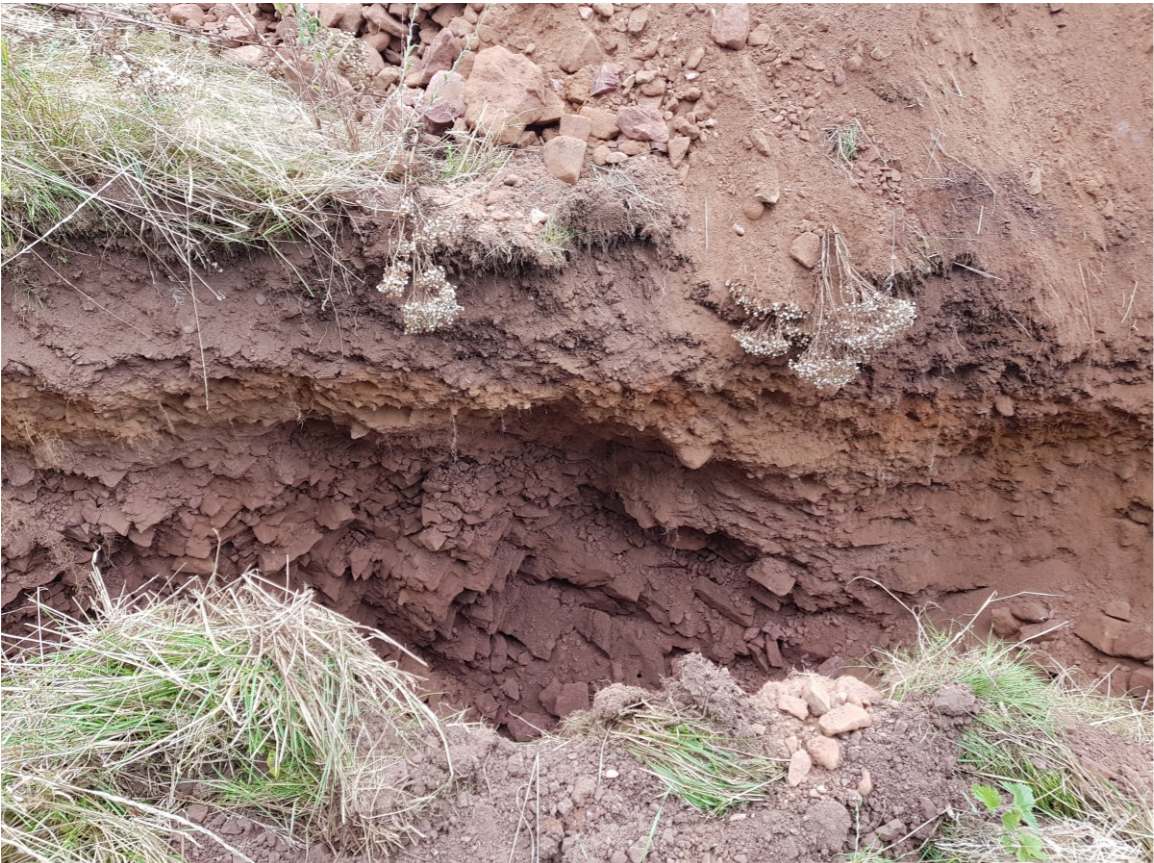
Number: TP09 Project Glounthaune Housing Phase 2 Project No P18170 Engineer AECOM
